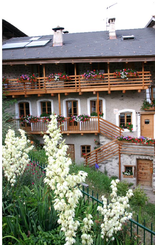
PICTURE 2. The refurbished building. Credit: Daniela Dal Bosco
