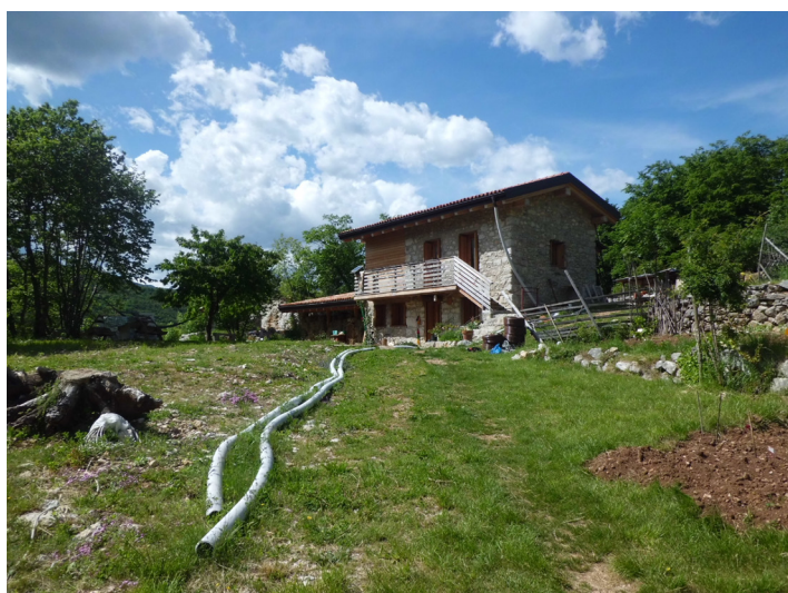
PICTURE 7. The building with the connection to the wetland plant. Credit: Floriana Romagnoli, Studio Vis
