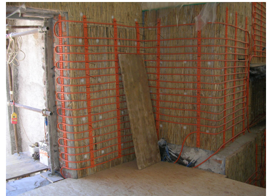
PICTURE 3. Tradition and innovation: wall heating associated with wattle and daub. Credit: Daniela Dal Bosco
